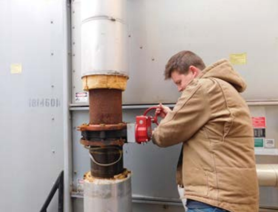
Photographed Above: Michael Brusic, Technical Director at Bright Power, testing out the new cooling tower isolation valves.
